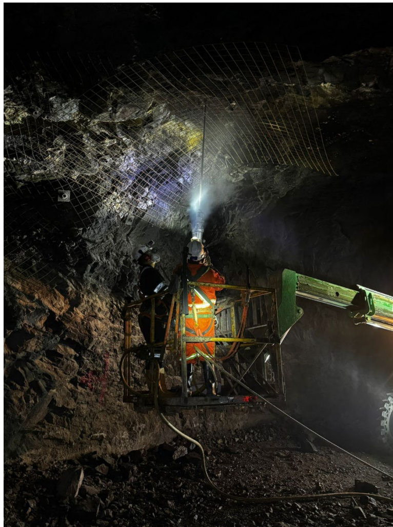
Figure 3: Installation of Ground Support at Promontorio
